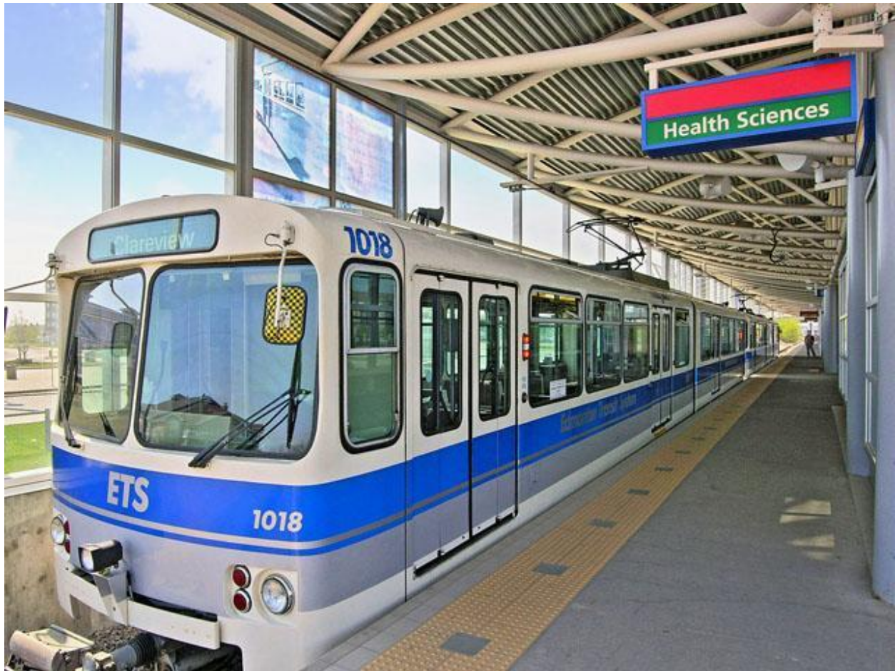
City of Edmonton South LRT Line, Health Sciences Station
