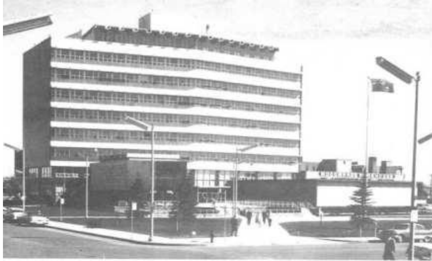
THE NEW CITY HALL EDMONTON, ALBERTA
